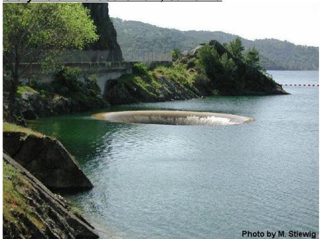
A glory hole is used when a dam is at full capacity and water needs to be drained from the reservoir. It is the largest spillway of this type in the world and consumes 14,400 cubic feet of water every second.
